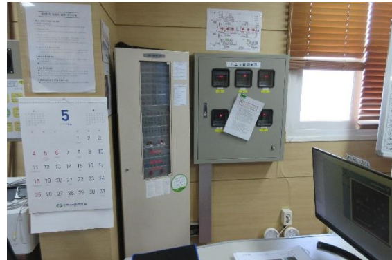
Fire control panel & Gas leak alarm
