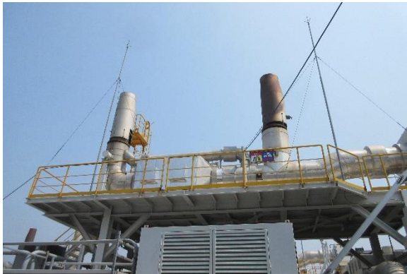
Lightning rod at the top of MCFC unit
