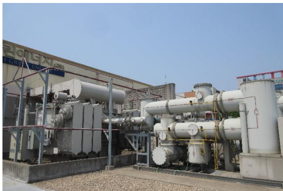
Main TRs & Switch gear
