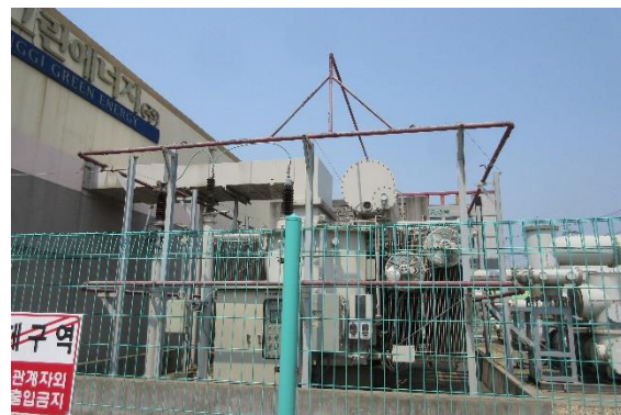
Water spray system for main TR
