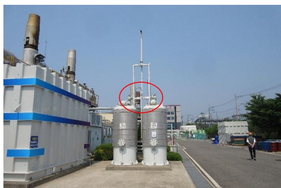
PSVs at the top of desulfurizer
